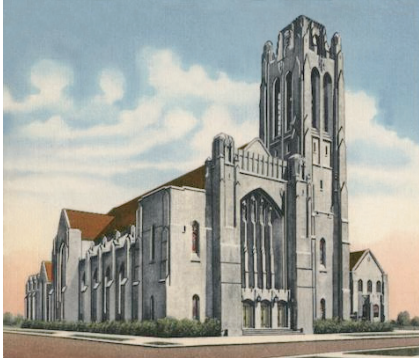
St. James Methodist Church Ellis Ave. at Forty-sixth Street Chicago 15, Ill.
